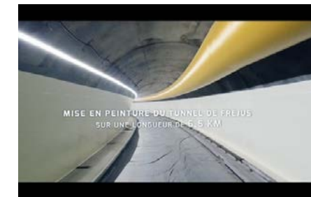
Revamping Tunnel de Fréjus
